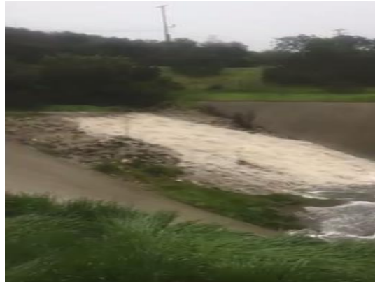
(Place curser over image, and hold down CTRL + click) Margate Canyon Creek Debris Basin PVDW at Apsley Rd handling storm water
